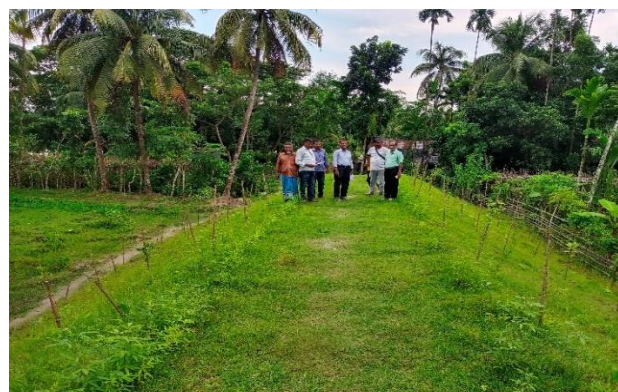
Figure 3-31: Embankment turfing and afforestation work at km 1+170 in Polder-39/2C
