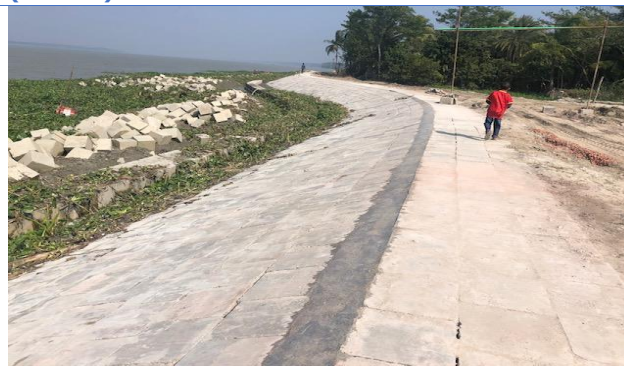
Figure 3-33: Slope & Bank Protection work in Polder-39/2C
