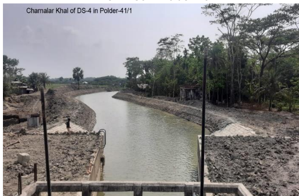
Figure 3-36: Completed DS-4 of Polder-41/1
