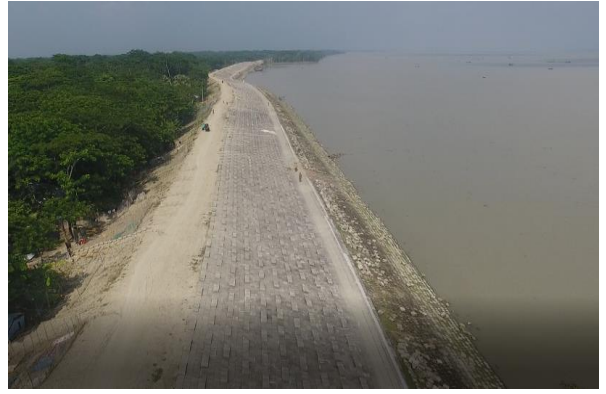
Figure 3-10: Completed Slope Protection Works in Polder-32
