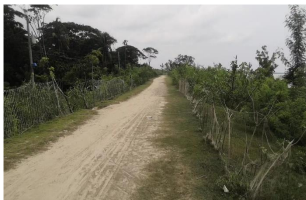
Figure 3-30: Turfing work for k13+100-k15+000 in Polder-40/2
