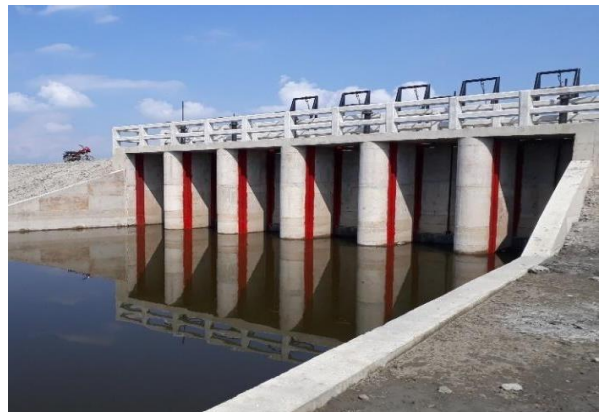
Figure 3-13: Completed 6 vent DS of Polder-35/3
