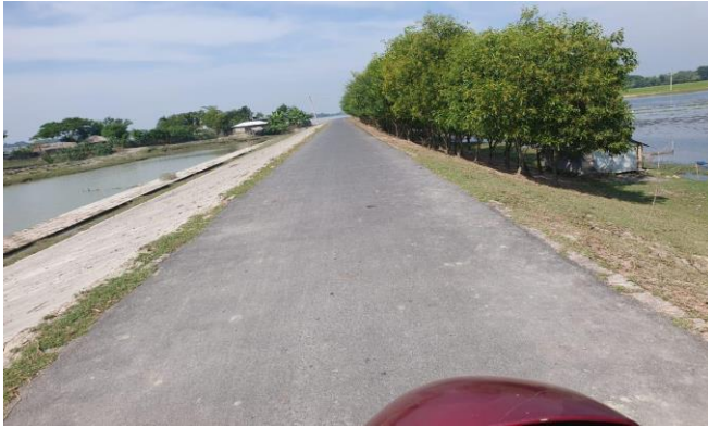
Figure 3-9: Completed Embankment of Polder-32
